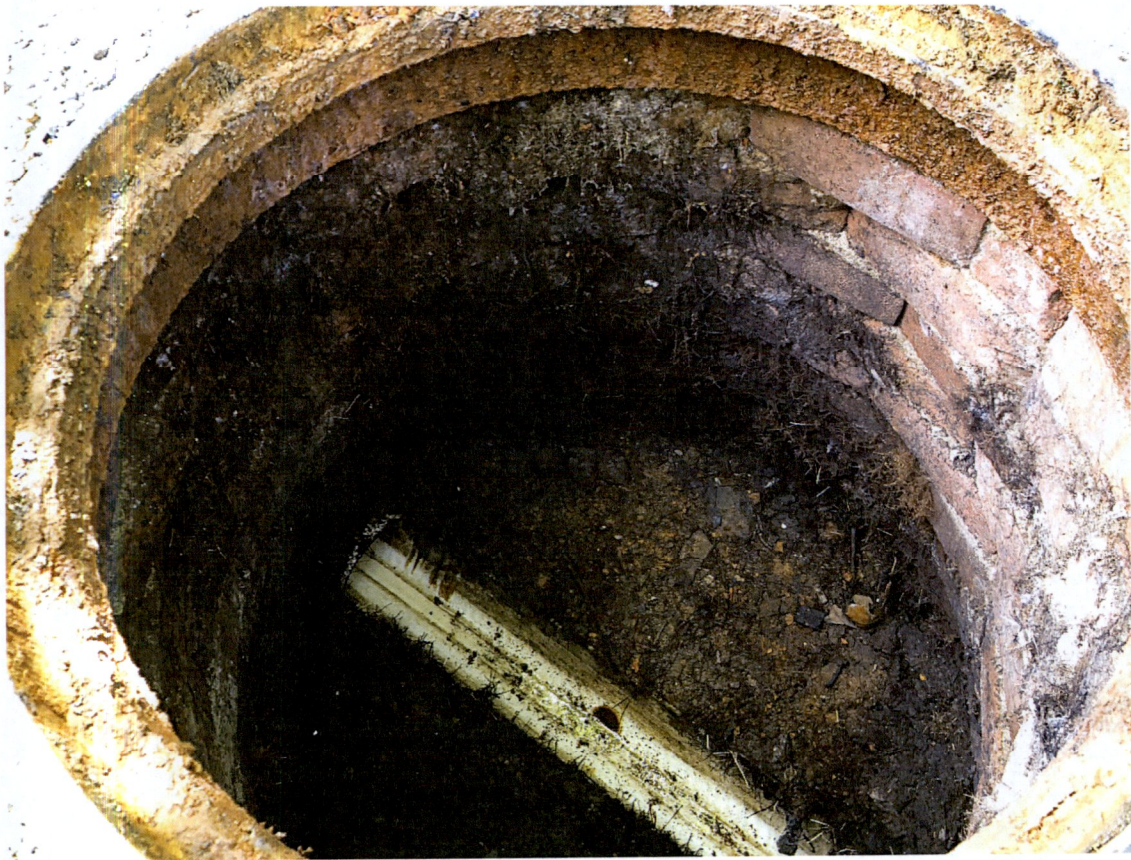
Brick Manhole Types in the Collection System (age and condition varies).
